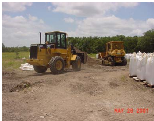
Figure 3. Mixing Apatite II™ into Lead-Contaminated Soil.
