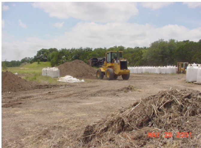
FIGURE 1. Soil mixing of Apatite II into Pb-contaminated soil at CSSA SWMU B-20.
