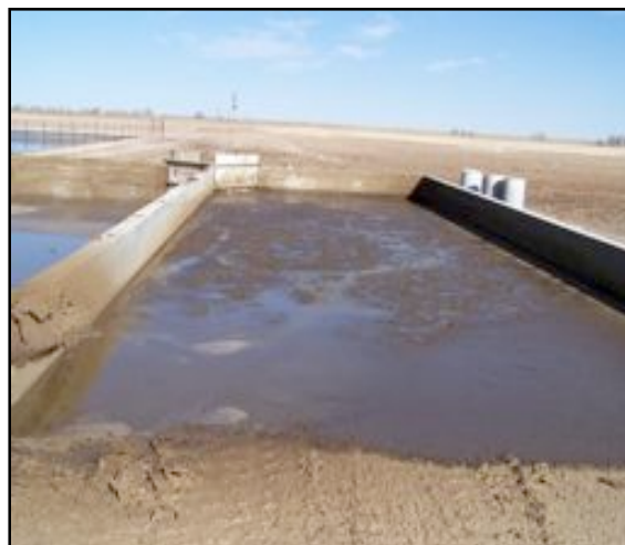
Figure 3. A solids separator prior to discharge into pond.
