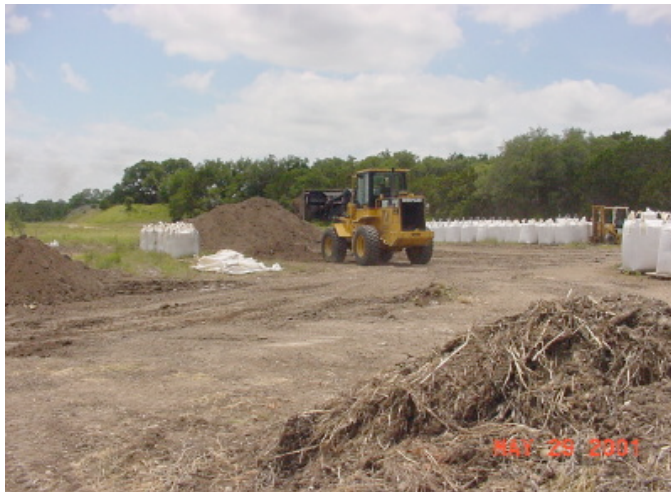
FIGURE 1. Soil mixing of Apatite II into Pb-contaminated soil at CSSA SWMU B-20.
